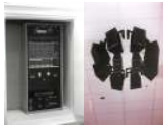
Colby College PA system installation.
