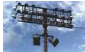
PA system installation at Sanford, ME high school football field.
